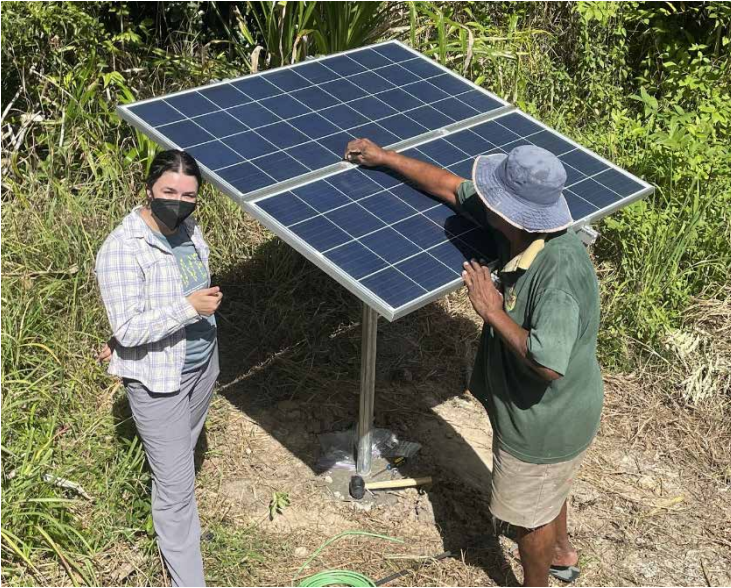
The Cal Poly Engineers Without Borders Fiji team worked on improving the quality and quantity of water in three rural villages in Fiji. Above: Work included designing a Vesi solar borehole pump system.
